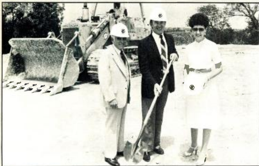
New digs. KTVU-TV Fort Worth has begun construction of its new $4-million studios (artist's conception above right). Above, General Manager Charles Edwards (center) turns the first shovelful of dirt, while Chief Engineer Walt Baxley (l) and Assistant General Manager Ocella Allison look on.
